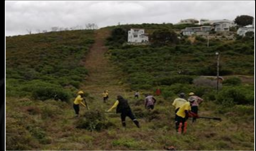
Fig 3: Mechanical firebreak construction (SCFPA 2023)
